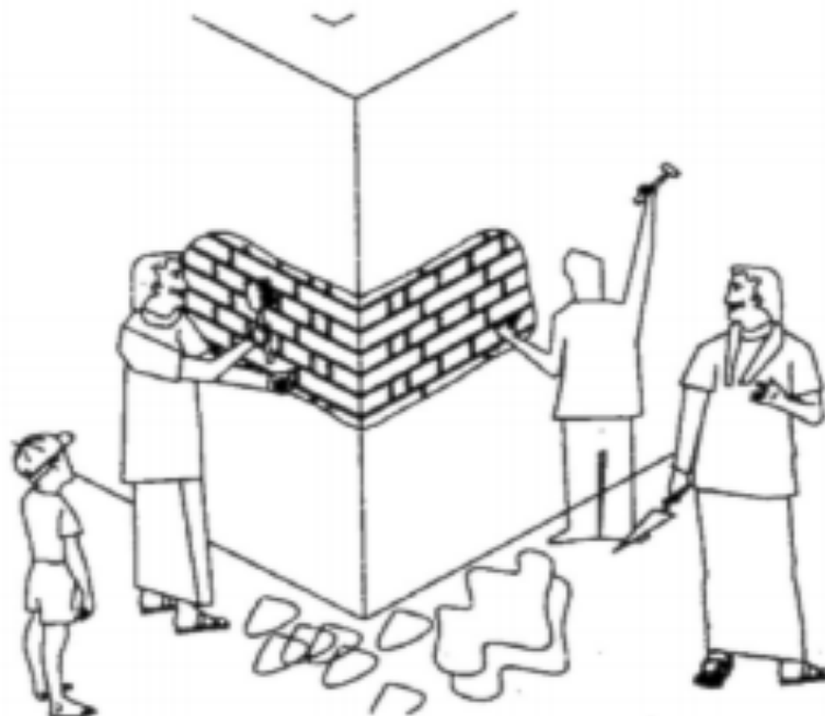
Figure 49: Removal of plaster and raking of joints process (Credit: www.btp.com )
