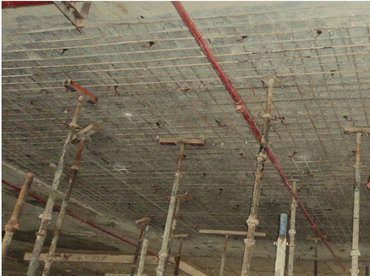
Figure 35: surfaces preparation for shot-crete (credit: researchgate)
