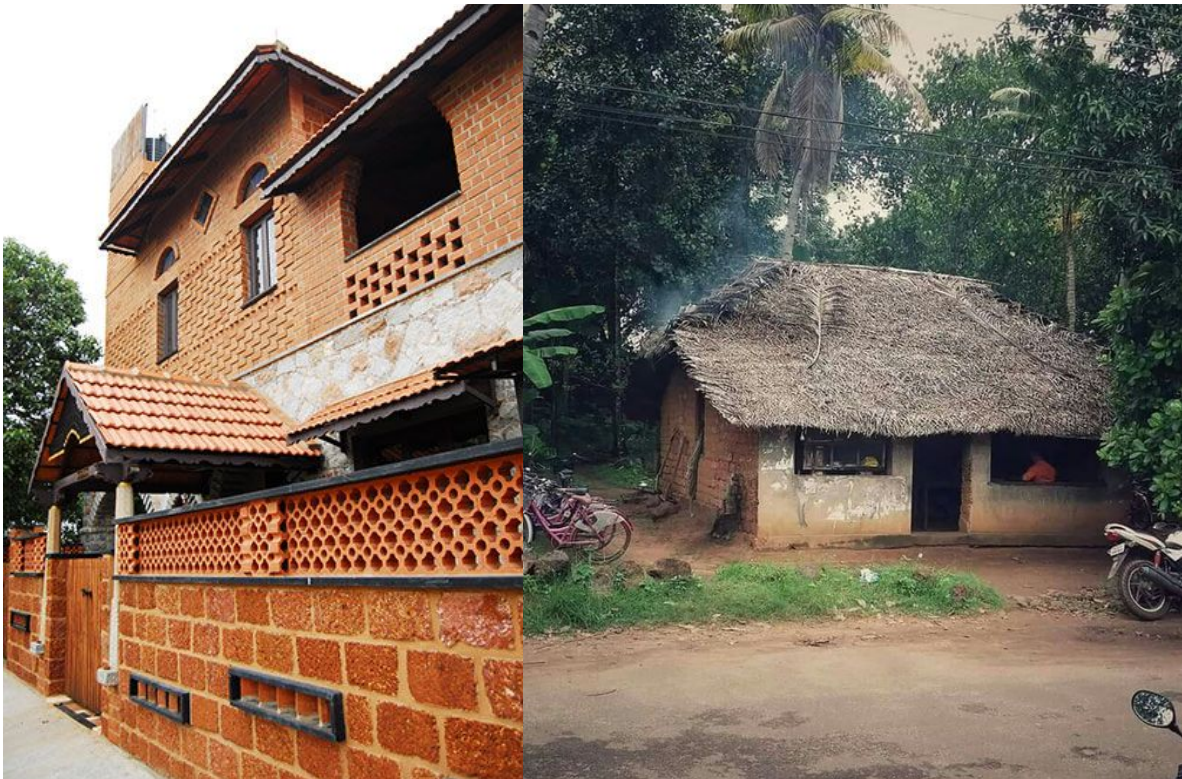
Figure 5: Image showing urban residential Building using laterite stone (left), typical rural residential building (right). (credit: pinterest.com)
