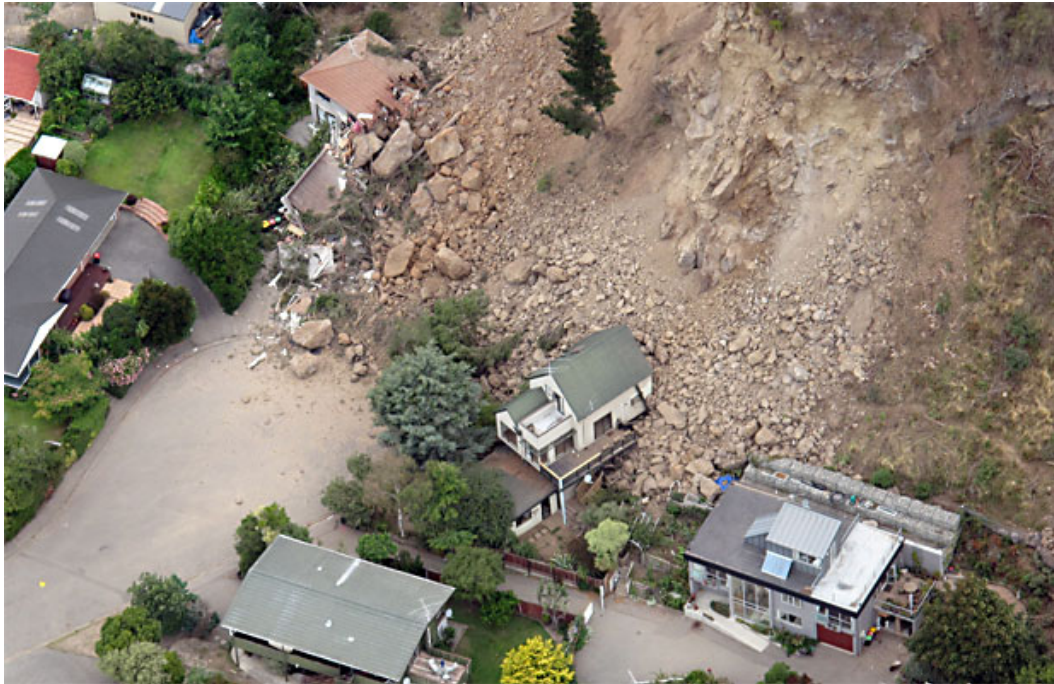
Figure 47: Building partially buried due to landslide (credit: http://www.stuff.co.nz )
