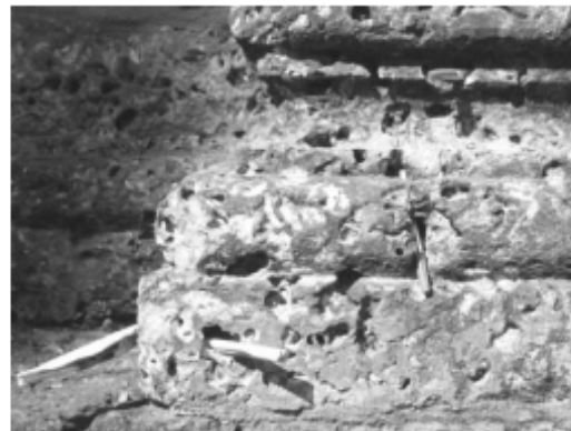
(b) Honey combing due to action of rain
