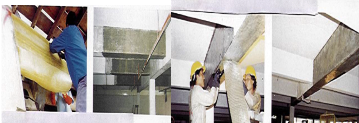
Figure 30: Jacketing of Beam using FRP (credit: TESRA ppt)
