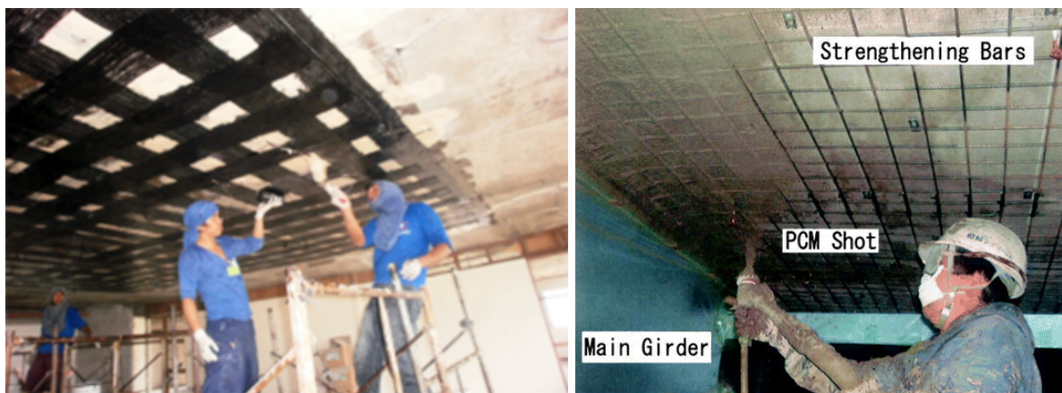
Figure 36: retrofitting using FRP (left) and shot-crete in slab (right) (credit: researchgate)
