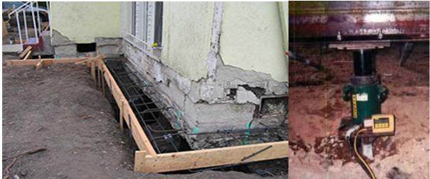
Figure 18: Image showing example of Retrofitting foundation using Jacks and extra reinforcement (credit: <u>www.renotahoefoundationrepair.com</u>)
