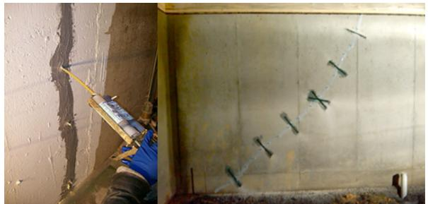
Figure 13:Image showing repair of crack using injection technique (*left*), repair of crack using diagonal bracing (*right*). (*credit: www.a1crackrepair.com*)
