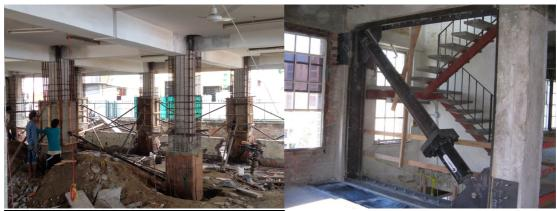
Figure 15: Images showing example of Retrofitting of basement (credit: urbansolutionsbd.blogspot.com)
