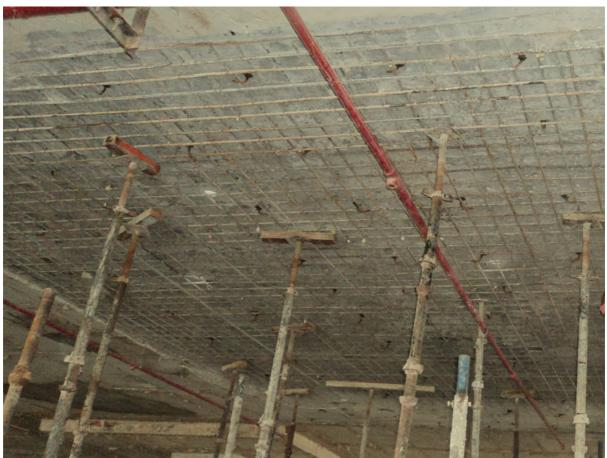
Figure 37: surfaces preparation for shot-crete (credit: researchgate)
