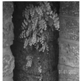
(a) Growth of moss and lichens Figure 53: Image showing damage due to bio-degradation in laterite stone (credit: iwww.hms.civil.uminho.pt)
