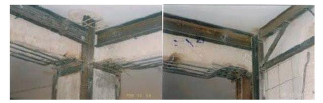
Figure 34: Strengthening a beam, slab & column (left) and Strengthening of beam and slab (right) (credit: researchgate)
