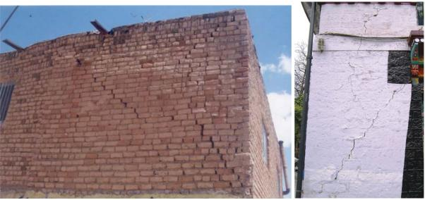
Figure 21: Image showing example of structural cracks in wall due to landslides (credit: ascelibrary.org)
