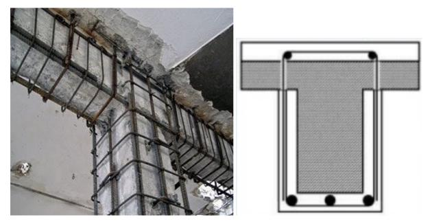
Figure 33: Jacketing of Beam using RCC jacketing (credit: yash construction)
