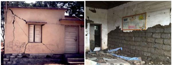
Figure 39: structural damage around opening (left) and damage due to flood (credit: http://db.world-housing.net)
