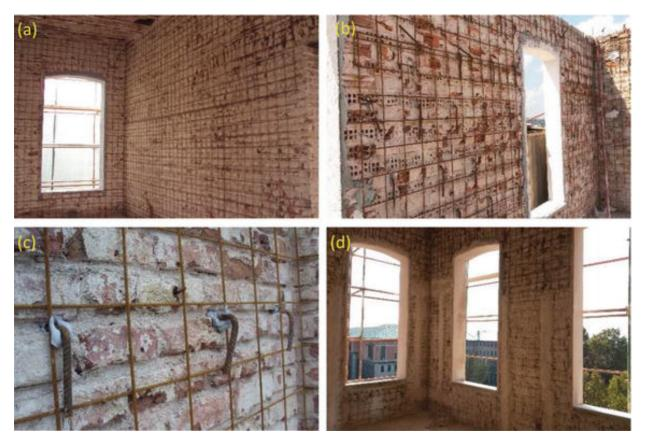
Figure 25: Retrofitting procedure of masonry building using iron bars (credit: www.intechopen.com)
