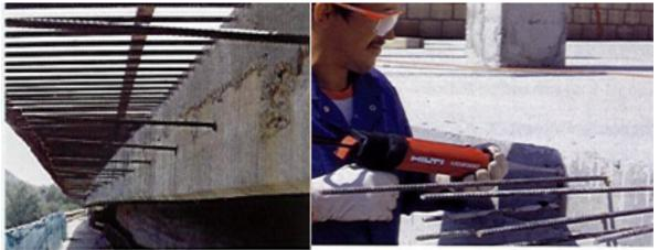
Figure 49: Re-bar fastening machine application (credit: TESRA ppt)
