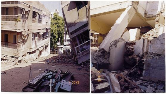
Figure 27: Collapse pattern due to soft story failure due to column failure (*credit: TESRA ppt*) **General retrofitting technique:** On the basis of damage assessment the result should be quantified, and Different retrofitting techniques should be adopted to rehabilitate the structure. if column is failing due to lack of concrete, then jacketing of column should be done. There are other several techniques are available for the retrofitting of columns as follows:
