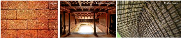
Laterite blocks Timber Thatch Weaving Figure 6: The images showing Construction Materials commonly used in Kerala
