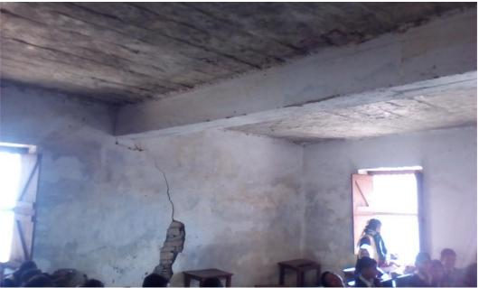
Figure 31: damage in wall and slab due to sagging (credit: daily civil)
