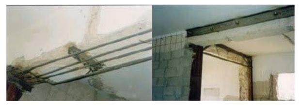
Figure 35: jacketing by bars in beam (left) and Strengthening by steel plate (right) (credit: researchgate)
