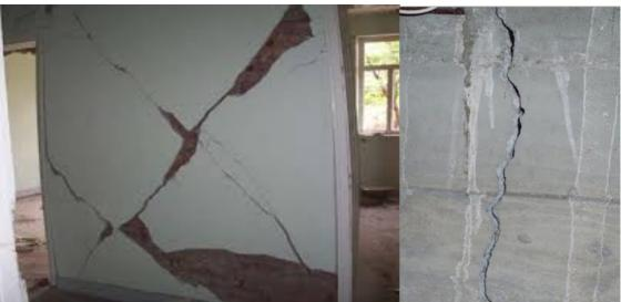
Figure 20:Image showing example of structural cracks in wall due to flood (credit: www.iitk.ac.in)
