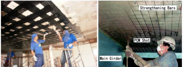
Figure 38: retrofitting using FRP (left) and shot-crete in slab (right) (credit: researchgate)
