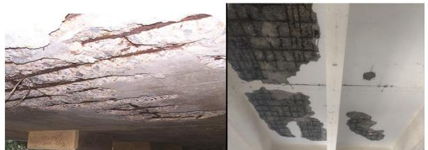
Figure 36: de-lamination and rusting in slab (left) and de-lamination of plaster in slab (right) (credit: researchgate)
