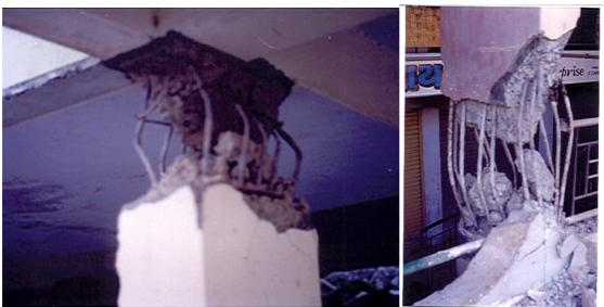
Figure 26: image showing damage in columns due to dynamic loading (credit: TESRA ppt)
