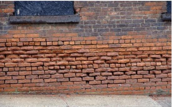
Figure 55: Image showing erosion of mortar due to flood water (credit: inspectapedia.com)
