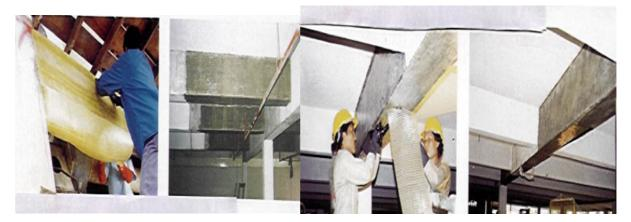
Figure 32: Jacketing of Beam using FRP (credit: TESRA ppt)
