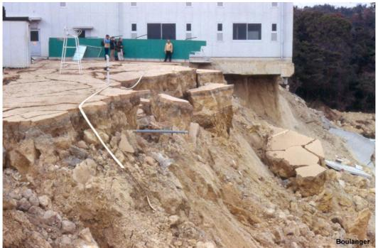
Figure 59: Base soil under foundation eroded due to landslide (credit: http://www.stuff.co.nz)
