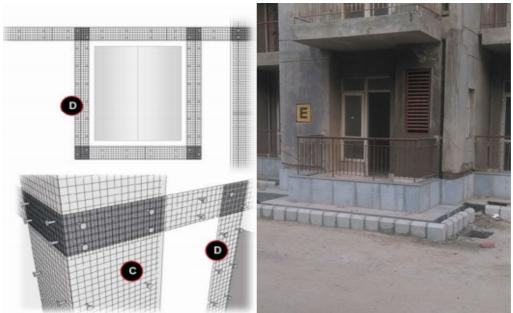
Figure 10: wire mesh installation for plinth protection (left) Stone plinth protection installation (right) (Credit: www.bptp.com)
