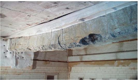
Figure 30: damage due to sagging (credit: daily civil)
