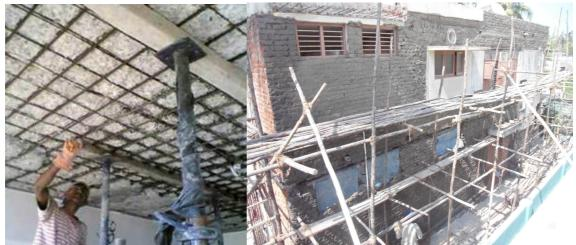
Figure 14:Image showing re-plastering and restoration of slab (*left*), Restoration process of front facade of building(*right*). (*credit: RMS civil repair works*)
