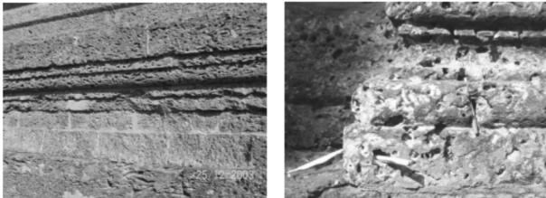
(a) Granular disintegration (b) Honey combing due to action of rain Figure 52: Image showing damage pattern in laterite stone (credit: iwww.hms.civil.uminho.pt)
