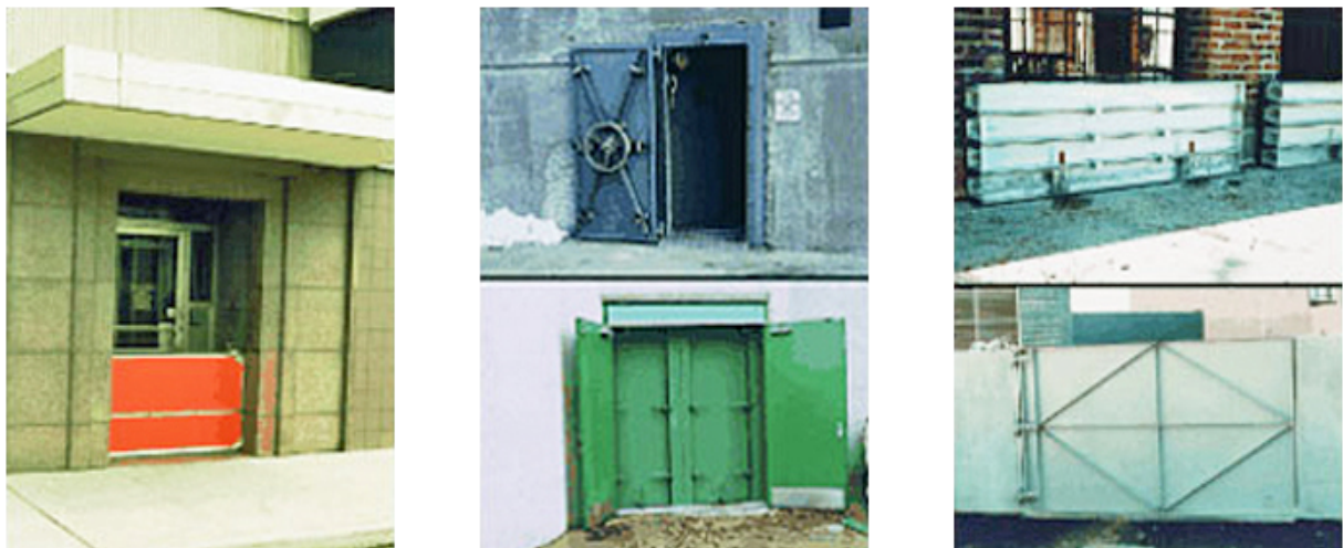
Figure 21: Temporary flood panels and permanent flood doors and gates (credit: andhitapradipta.github.io)
