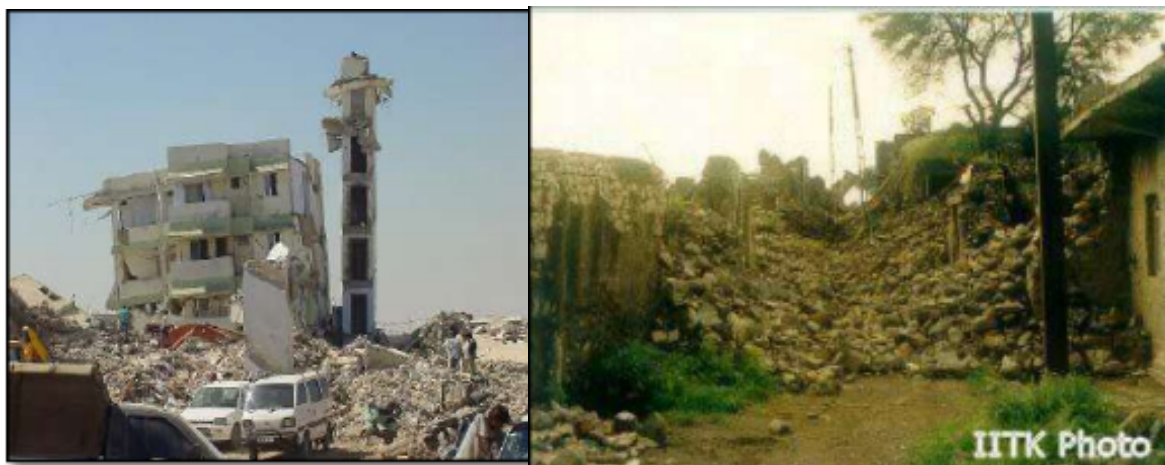
Figure 14: Apartment collapse in 2001 Bhuj earthquake with separation of the lift shaft (credit: IITK)
