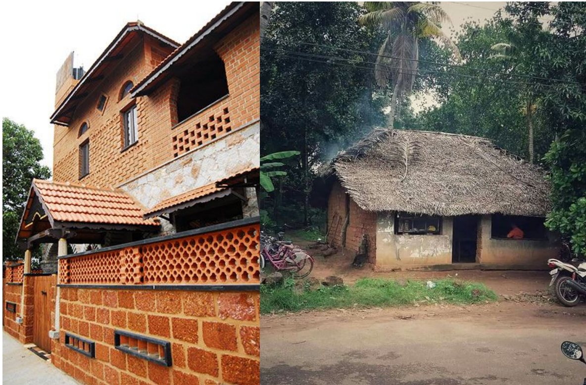
Figure 7: Image showing urban residential Building using laterite stone (left), typical rural residential building (right). (credit: pinterest.com)
