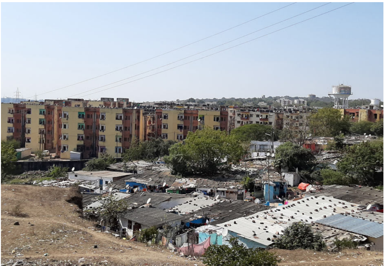
Image 4.7: EWS housing blocks under the RAY scheme in Nehru Nagar on the banks of Upper Lake
